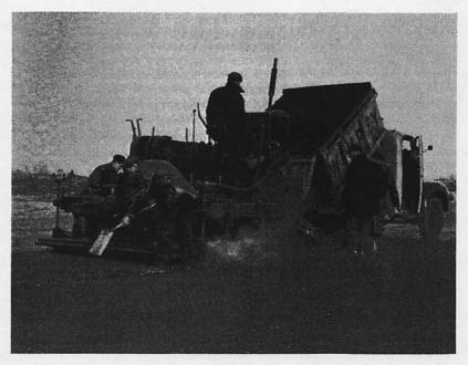
The construction of runways on the South Airfield proceeds steadily, though much remains to be done. Here, one of the machines involved in the work can be seen laying asphalt
