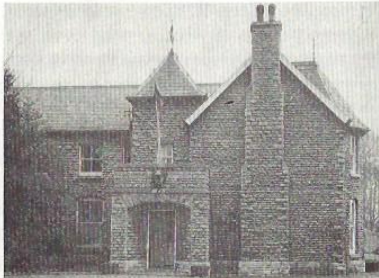
A view from the South showing the original building and extensions.
