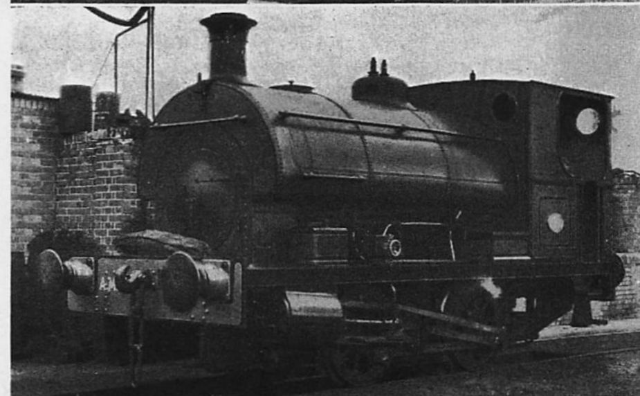
A.M.W.D. No. 127, Peckett 0-4-0 saddle tank at Cranwell, May 1953. A sack of coal is carried on the buffer beam in case the limited bunker space is insufficient on any journey
