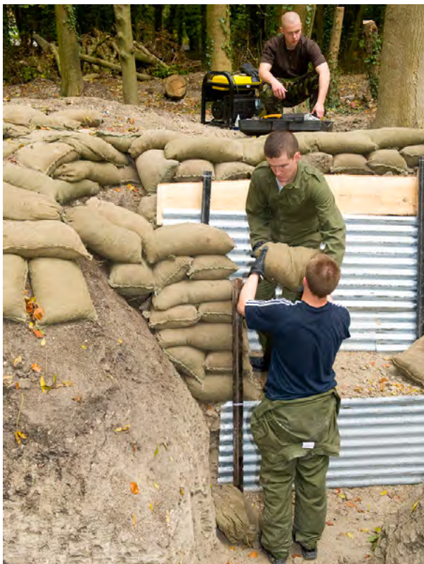
SATTs helping restore the WWI trench at RAF Halton.
