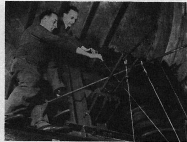
Messrs Allsop and Mooney, of Gent and Co., Ltd., adjusting one of the many operating cables connecting the hammers with the striking mechanisms
